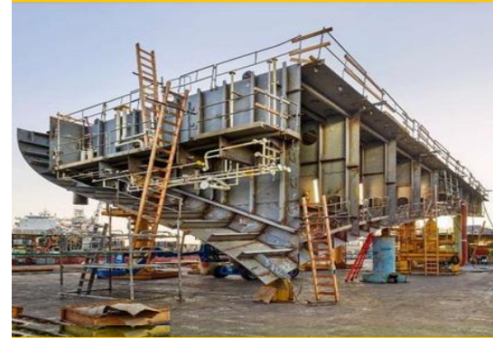
Launching Steel Girders
